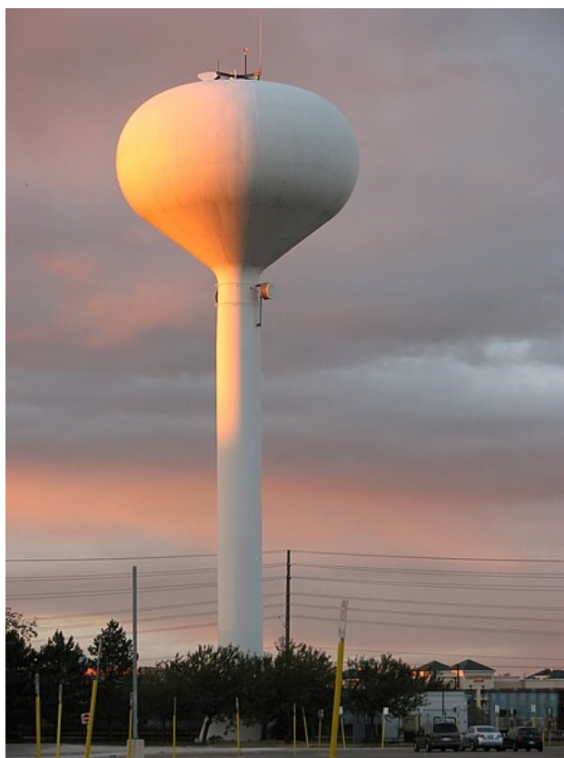
A typical municipal water tower holds 1,000,000 gallons of water image: Wikipedia
